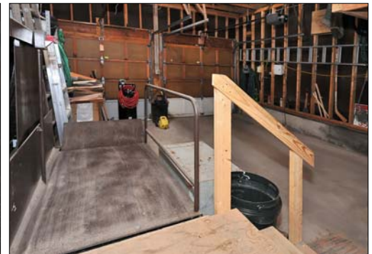
PLATFORM LIFT FROM GARAGE
